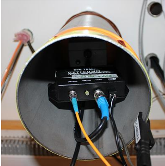
Image 13. Filter box (on the back) and optic transmitter (on the front) inside the waveguide.
