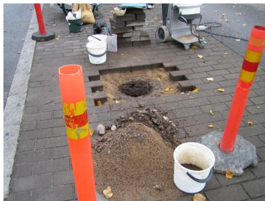
Picture 1. Load-bearing planting soils are expensive to sample later on, as they are paved over. Pavement must be removed to access the soil below. Soil augers do not penetrate the stony mix and any sampling must be done by digging soil pits. Image by Anu Riikonen.
