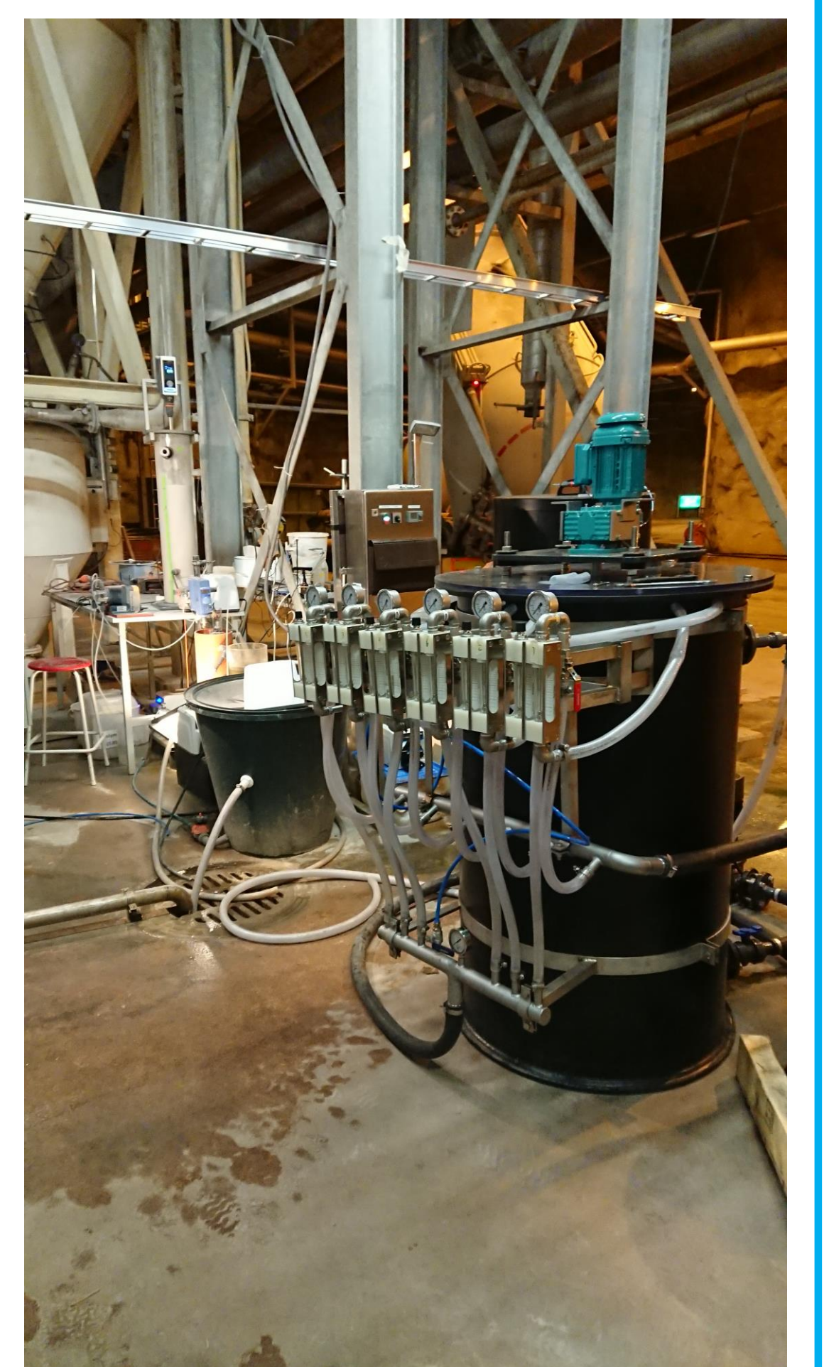
Figure 4: Piloting area in Viikinmäki WWTP.
