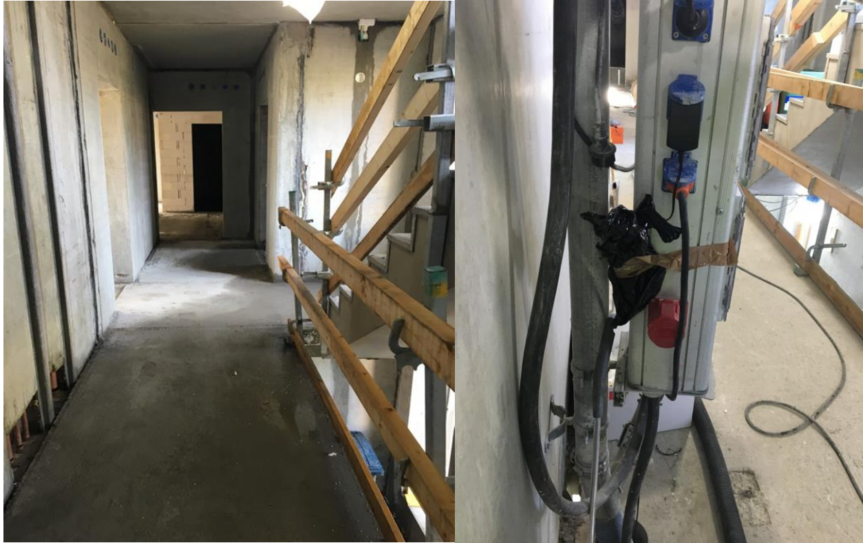
Figure 23 Onsite conditions (left) and gateway attached at the power supply each floor (right)
