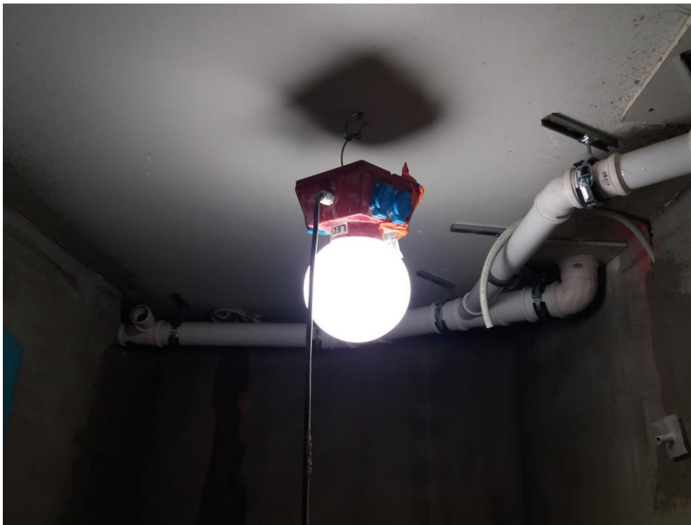
Figure 13. Gateways attached on the construction lamp onsite
