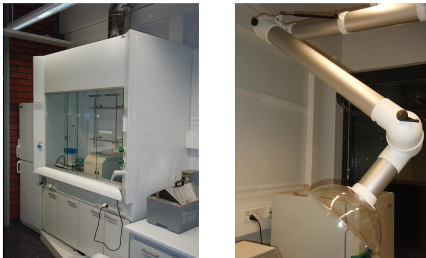
Figure 21 Vapour hood and local exhaust ventilation
