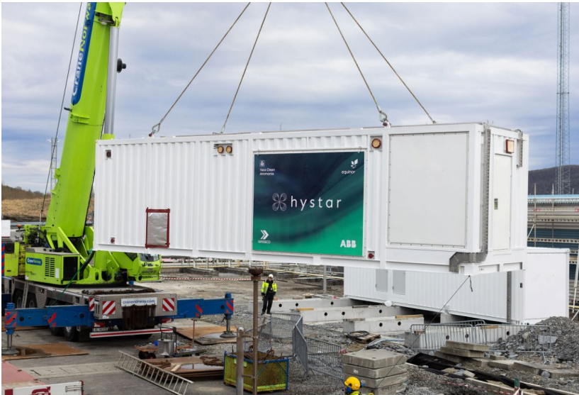
Hystar PEM electrolyser container in Equinor's site in Norway
