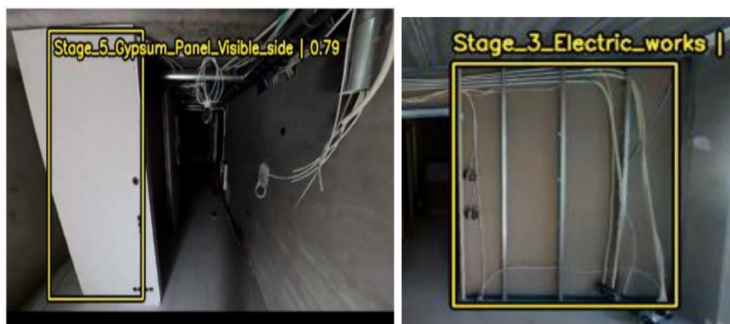
Figure 17: Detection of visible side of gypsum board and electrical work stage
