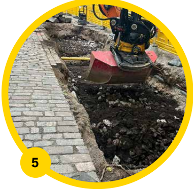
5 Structural soil renovations (17m 3 )
