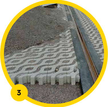
3 Tram rail roads with green paving stones (9.25m 3 )
