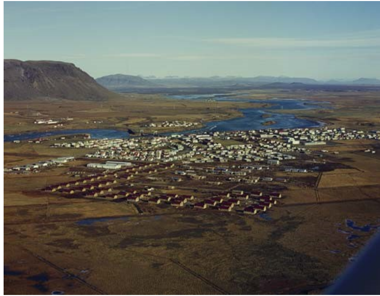
FIGURE 3.5 Aerial photograph of Selfoss, South Iceland, in 1974, featuring the recently implemented Vidlagasjodshus in the front. Credit: With the courtesy of the photographer Mats Wibe Lund.
