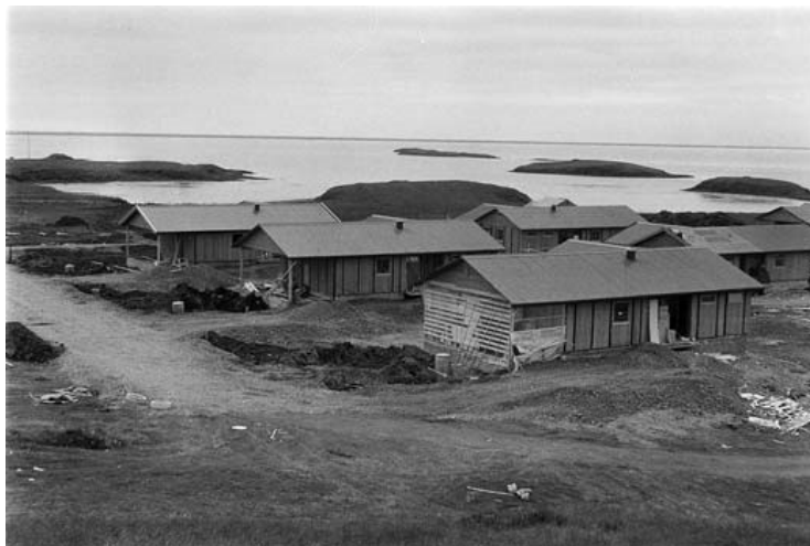
FIGURE 3.4 Disaster-relief houses under construction in Höfn, South Iceland, in 1973. Credit: Photography by Vilborg Harðardóttir, with the courtesy of The National Museum of Iceland.
